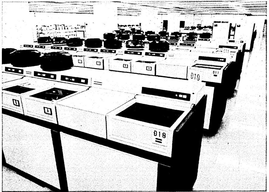
Foreground unit labeled D10 is the cross-call adaptor devised to assure fail-safe operation of peripherals.
