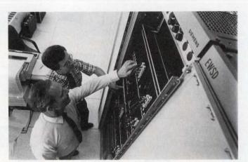
For testing ISDN equipment and services, the Advanced Technology Laboratory at Southwestern Bell Telephone in St Louis contains four digital CO switches, including this Siemens EWSD.
