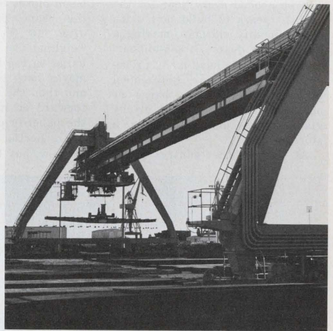
Eventually this gantry will use a computer-made tape, instead of an operator, to pick up steel panels from barges that come up the Pascagoula River to Litton's yard in Mississippi. It will be programmed to put them in the right piles.
