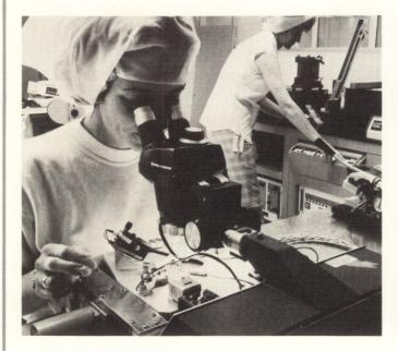
Before production gets under way, the "raw" wafers must be inspected for flatness, and for crystal dislocations and resistance in ohms per square centimeter.
