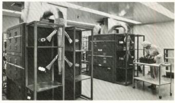
**Diffusion Temperature Check** Temperature of tube diffusion zone is spot-checked before loading with wafers.
