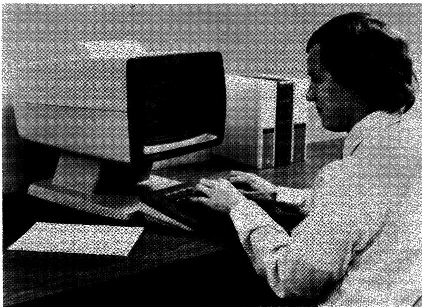
Hewlett-Packard's 2620 Series of display terminals provide the user with a wide variety of functions and capabilities. The 2621B, shown here, is the low-end model of the series. The 2621B is a character-mode smart terminal featuring two full pages of display memory. The integral thermal printer, contained in the 2621B's display case, is optionally available on all models in the 2620 Series.
