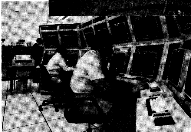
A 24-hour manned control center monitors on-line computer operations.
