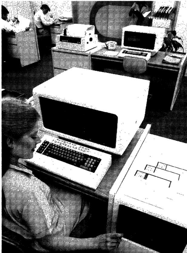
*The 5280 Distributed Data System is a diskette-based DDP system designed for applications such as intelligent data entry, batch and interactive communications, batch processing, and transaction processing. A variety of software is available for the 5280 system, including 3270 emulation.*
