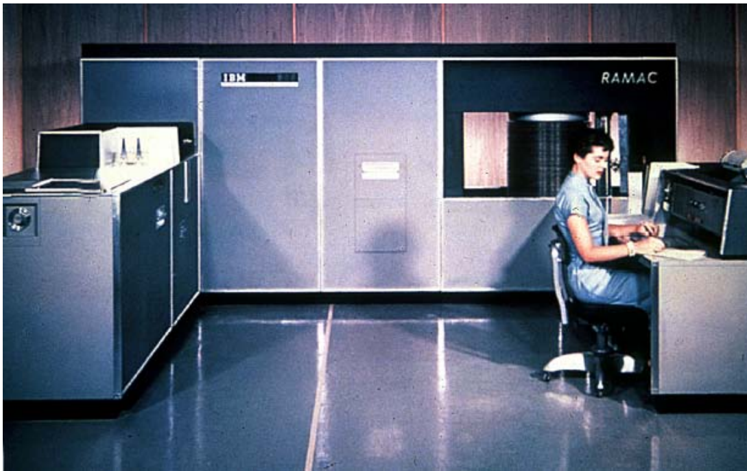
IBM RAMAC 305 Computer System, 1956
