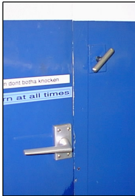
Figure 60 Safety Circuit Door Handle & Lock (In the locked position)
