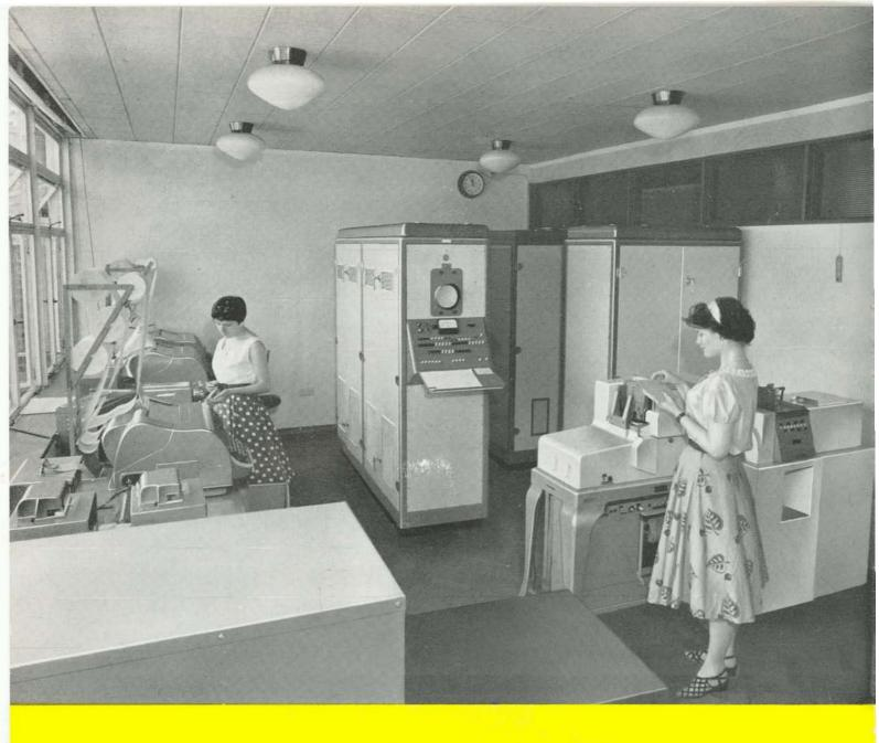
A double input-output Stantec-Zebra computer used for transonic and supersonic aerodynamic research at the Aircraft Research Association, Bedford, England.
