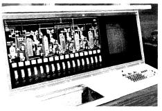
Fig. 3. This panel is in the pulp mill digester house at Great Southern Paper Co. in Cedar Springs, GA. It is  $19'' \times 43''$ , not including the crt display, and contains 342 lights.
