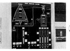
Fig. 1. At Mead Paper Co. in Escanaba, MI., the Bark Boiler panel is 36'' x 42''. It displays 38 pilot lights and 10 meters, in addition to 3 pushbuttons, 6 selector switches, and 6 rheostats.
